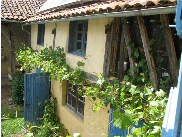
RISCLE ECO CONSTRUCTION
