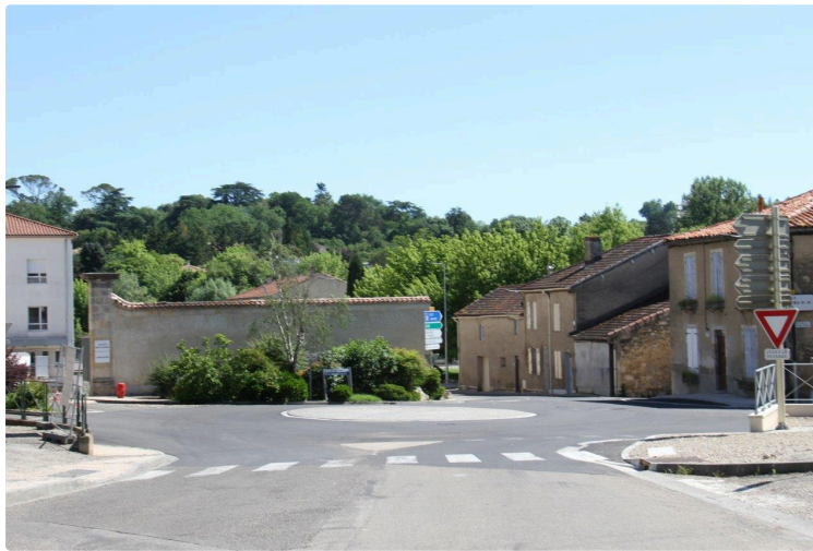
Travaux rond-point place Raymond Castaing
