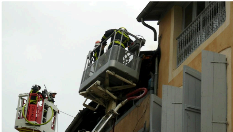
Important incendie rue Mirabeau
