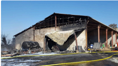
pompier gaz oil 3.JPG
