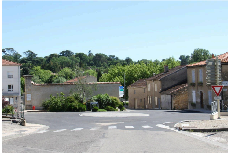
Travaux rond-point place Raymond Castaing
